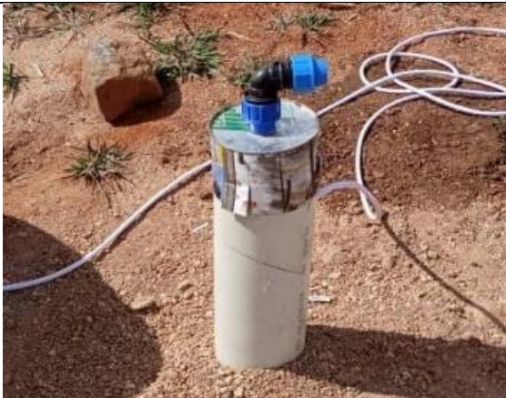
Cover the borehole
