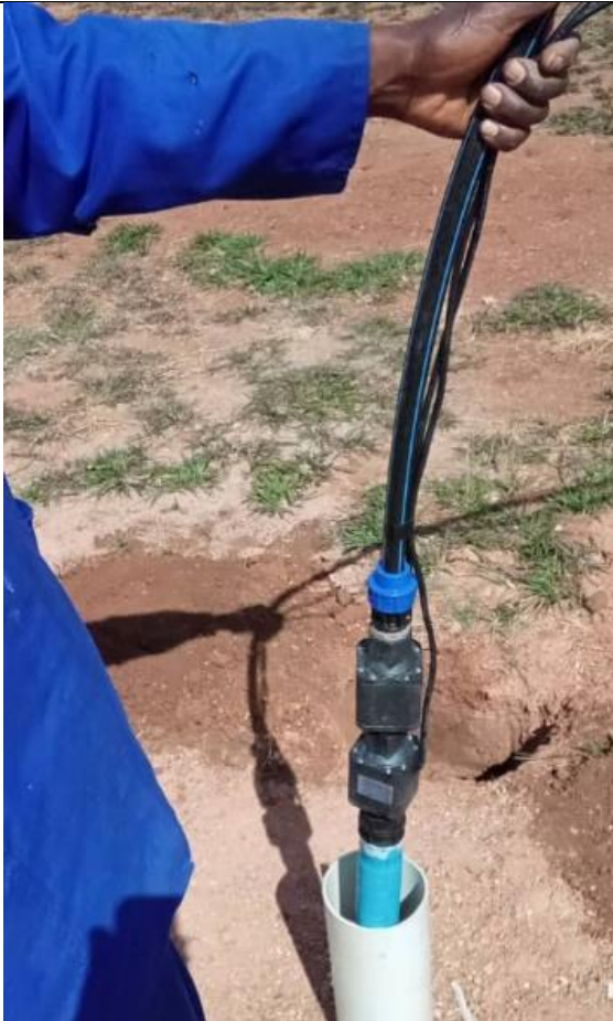
Installation in a casing of 90 mm
