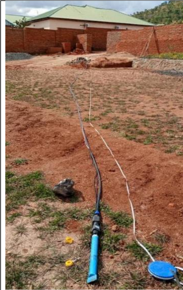
Installation of 2 pumps model ZL 50-20N
