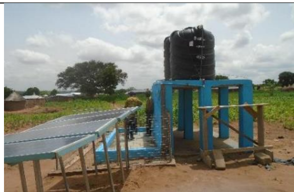
4 pumps ZL50-20N in series powered by 4 panels of 100 Watt. Water is used for communal water supply
